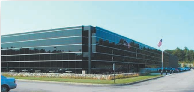
Pollak's® Canton, Massachusetts manufacturing plant.
